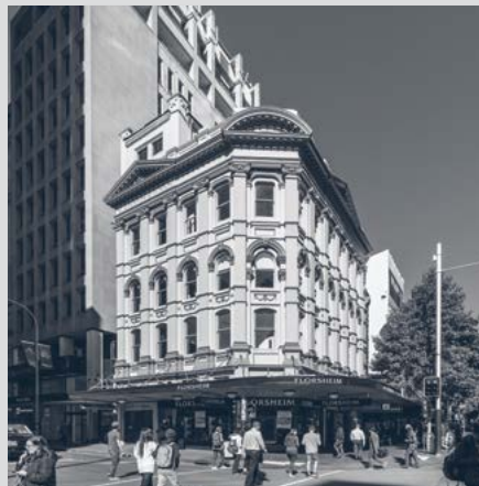
BLACKETTS BUILDING AUCKLAND CBD $21,750,000
